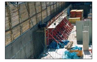
In addition to its primary drainage function, Enkadrain CK 20 has in this project been serving as a flexible separation layer.
