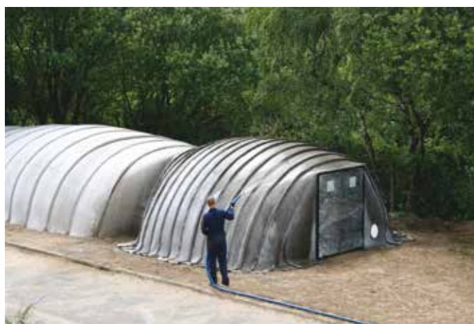
2. I Concrete Canvas Shelter
