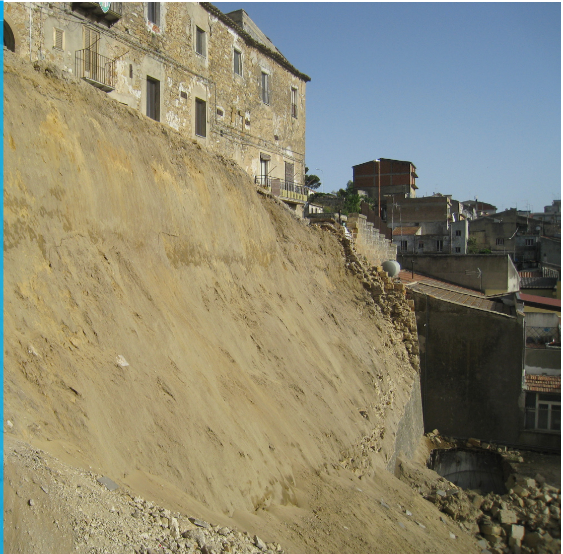
The slope prior to installation
