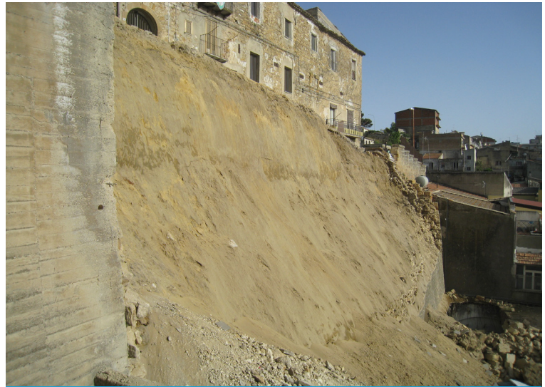
The site following the wall's collapse
