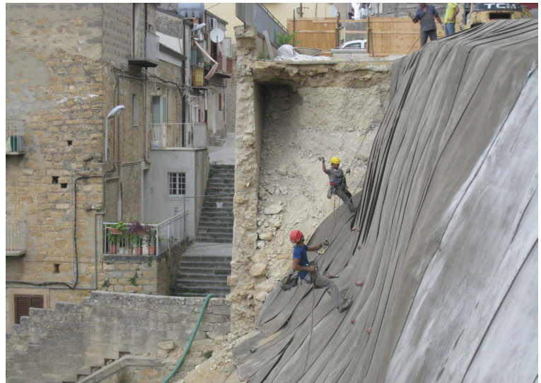
Two rock climbers assisted on the installation
