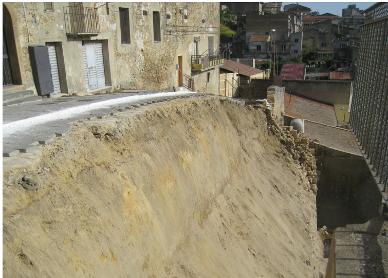
The wall's collapse also took down some of the carpark above
